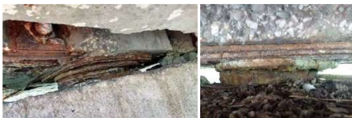
Figure 12 Corrosion of bearing and its deflection by the displacement of the superstructure
