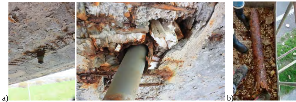
Figure 6 Detail of drainage pipes (a); original steel pipe after falling from polystyrene filled gap in lower flange (b)
