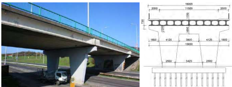
Figure 2 View of the bridge(a), bridge cross-section (taken from the bridge notebook)(b)
