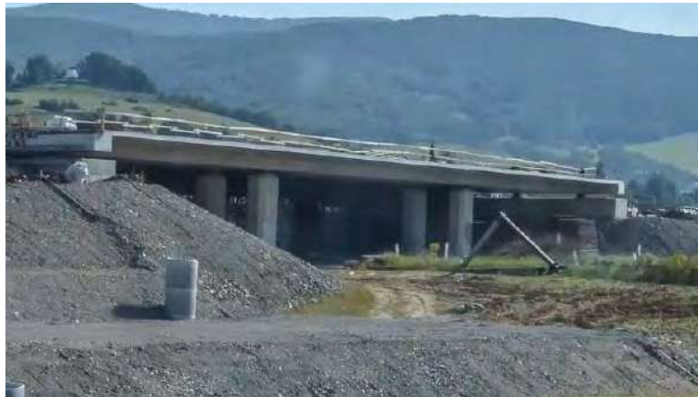
Obr.7 Most na R2 nad III/2632 v km 10.500
