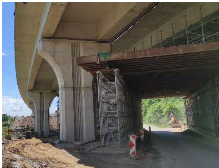
Obr.9 Most na R2 nad III/2664 v km 15.400
